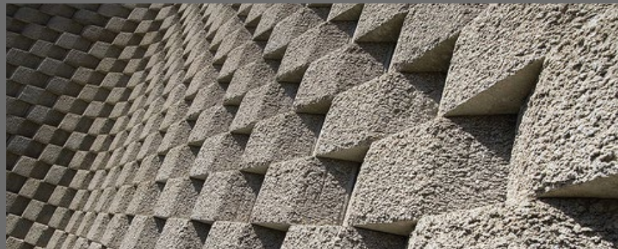
RE WALL BLOCK BRIDGE
